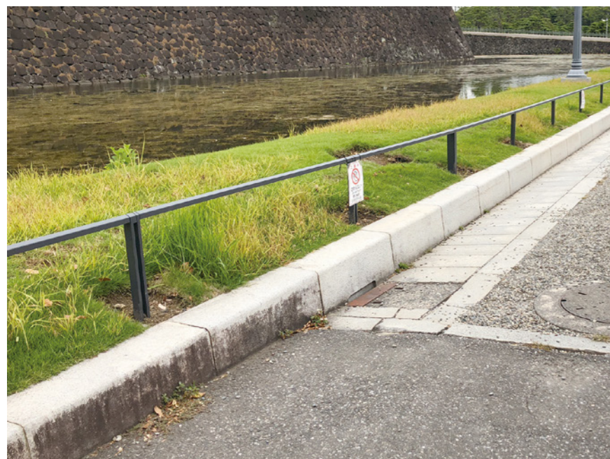
左側は施工前、右側は施工後
